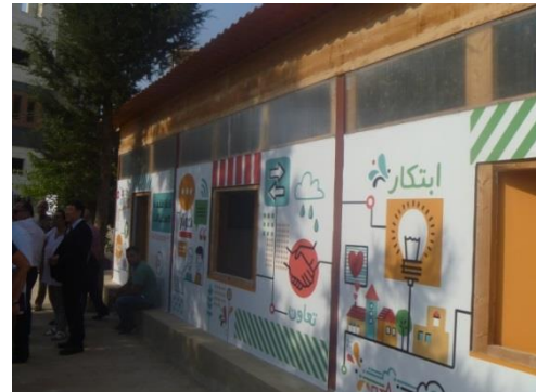
Multipurpose Hall at the Community Center
